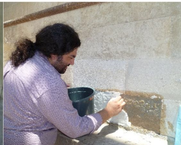
Fig. 26. Blasting and salt cleaning of cement imitations
