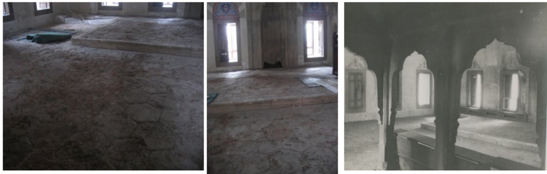
Fig. 23. Brick flooring emerging under the screed (left), brick floor in front of the mihrab (middle) (8) and photograph of the mosque flooring before the repair in 1936 (right) (6)
