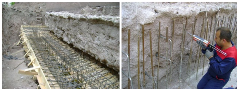
Fig. 14. Cap beam formwork and reinforcement and concrete manufacturing (left) and anchor manufacture (right) (8)
