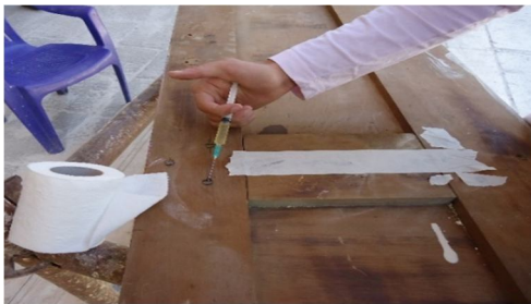
Fig. 25. Conservation of the wooden entrance door
