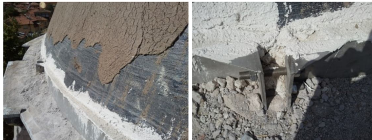
Fig. 15. Blasting with stainless tensioning application and silicium (left) and joint bolts (6)
