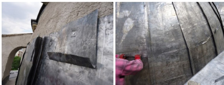
Fig. 16. Making lead covers, 2011 (8)
