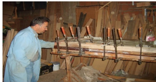
Fig. 25. Conservation of the wooden entrance door
