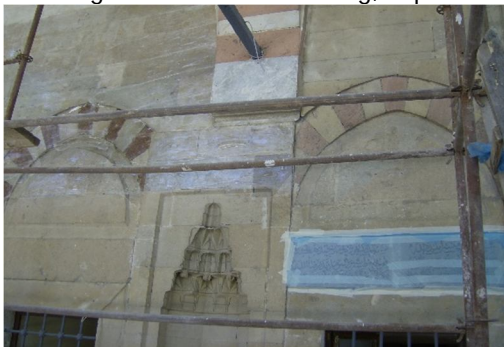
Fig. 27. Cleaning and protective application on exteriors
