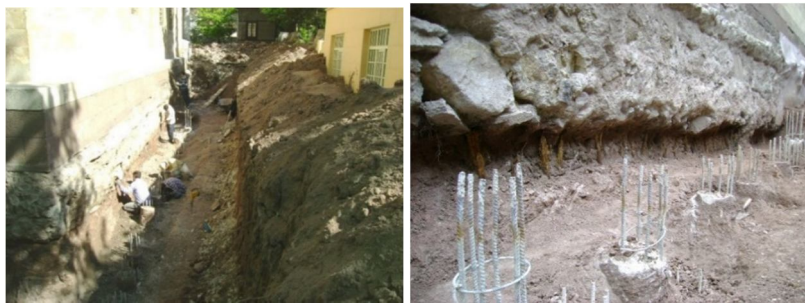
Fig. 13. Excavations and wooden piles that emerged in the meantime and newly manufactured mini piles, 2010 (8)
