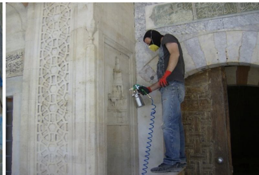
Fig. 27. Cleaning and protective application on exteriors
