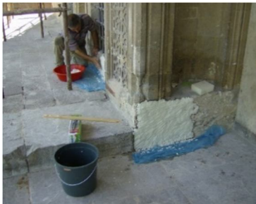
Fig. 26. Blasting and salt cleaning of cement imitations
