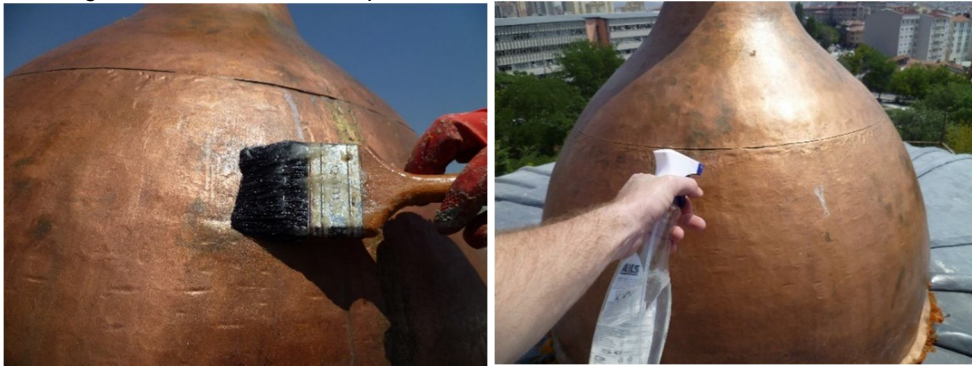
Fig. 28. Cleaning and protecting of copper finials
