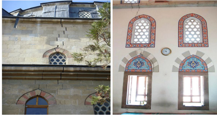
Figure 10. Structural crack exterior and interior view (8)
